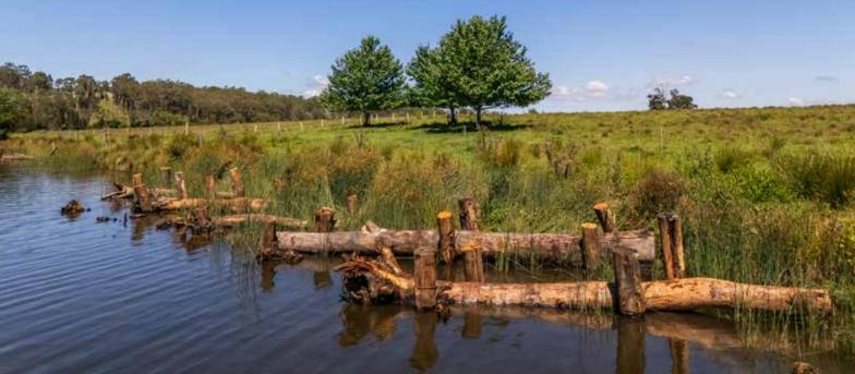
Hunter Water is working to stabilise eroding river banks on the Williams River, between Seaham and Clarence Town, to help prevent further erosion and improve water quality.
